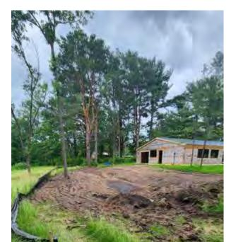
Rain garden over excavated awaiting backfill with soil media. Discussed bluestem on the side slopes, and plantings with 12-18" spacing in bottom. Discussed adding tile tube to gutters to ensure roof runoff from east end reaches the garden.
