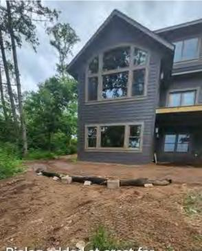
Biolog added at crest for additional protection. Discussed covering all soils with straw mulch and adding row of silt fence tonight before storm.
